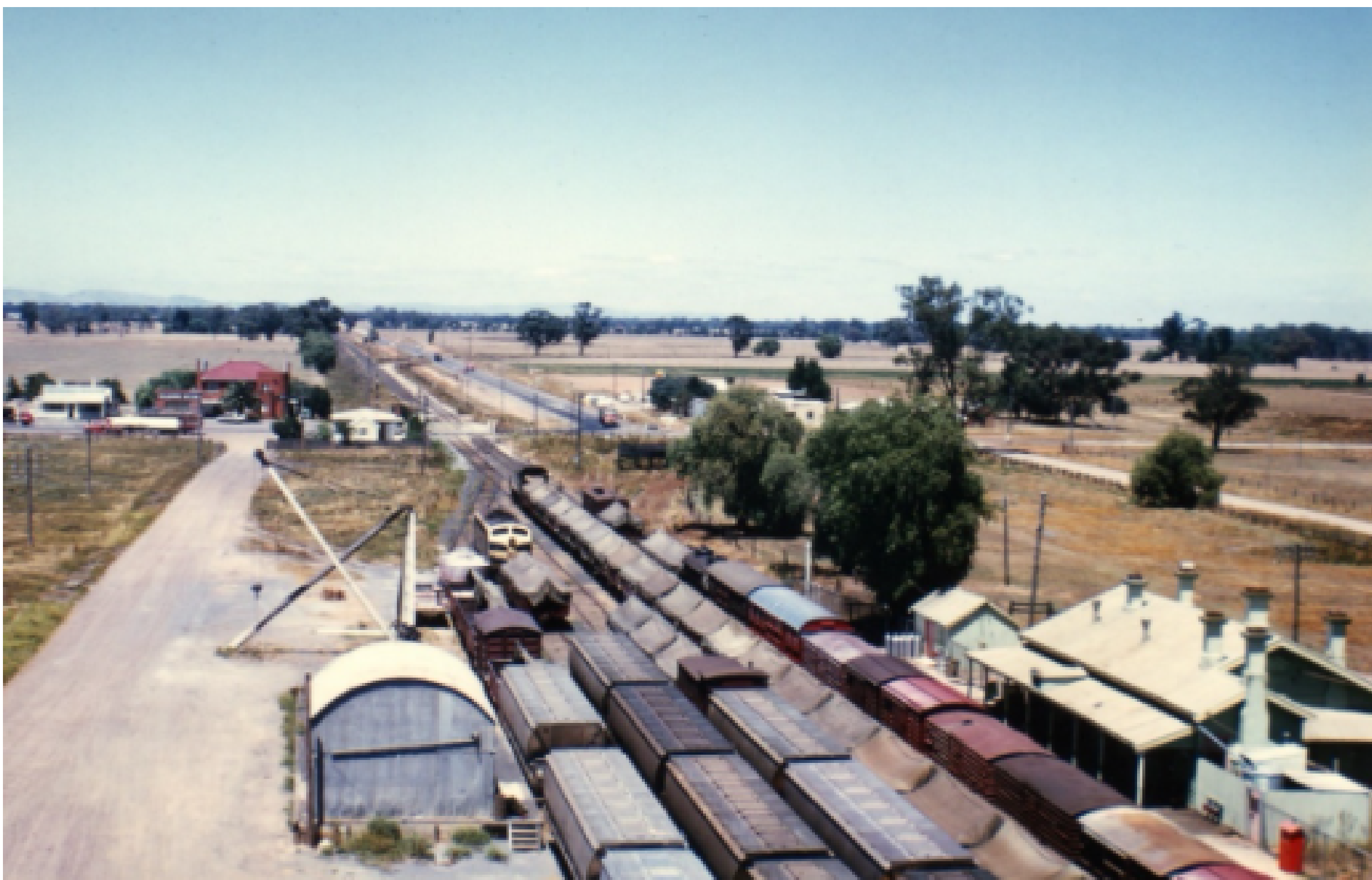
Murchison East railway station with goods trains transporting goods 1968 © M&DHS Inc. Wooden hand operated gates at road crossing (replaced 1974), gate-house for gate-keeper and track of branch line to Rushworth can be seen in the distance.
